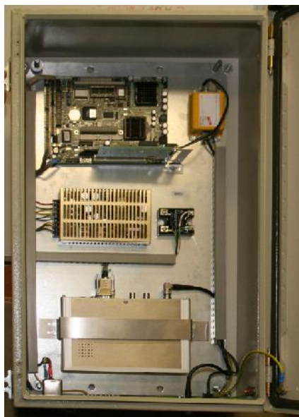
Onderstation FM monitoring
